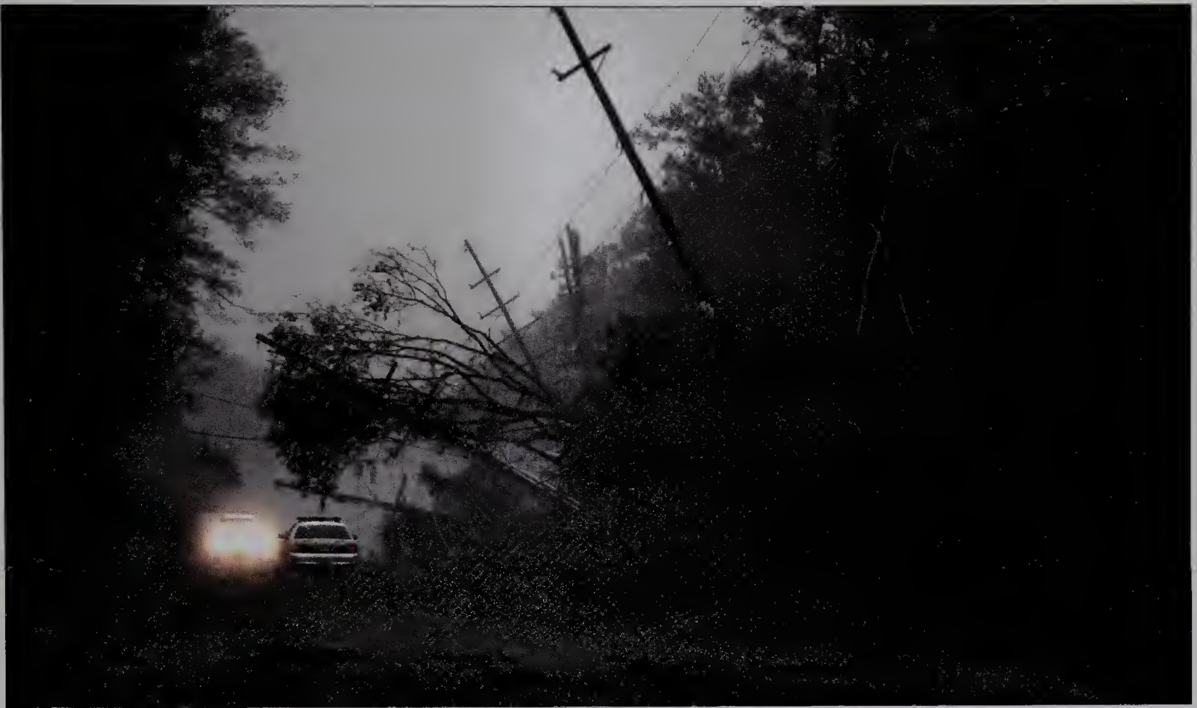
Broken utility poles, Mandeville, LA
